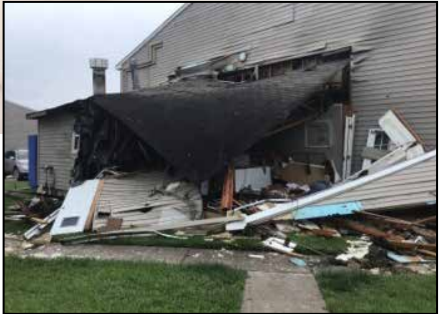
Figure 4 – Low Order Explosion Damage
