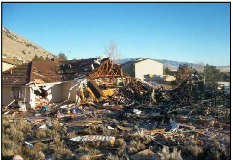
Figure 5 – High Order Explosion Damage
